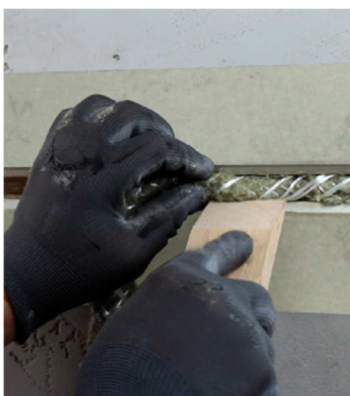
Vložte provazec Nullifire FJ203 do spáry.
